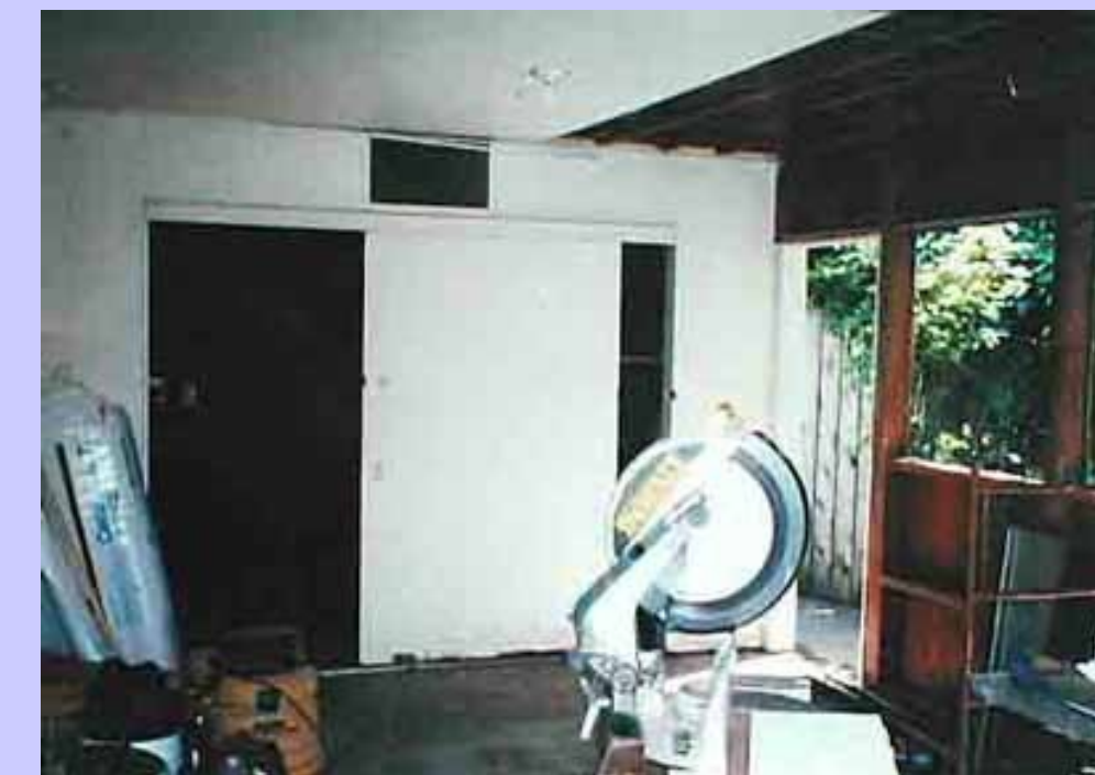
Carport south wall, 2000
