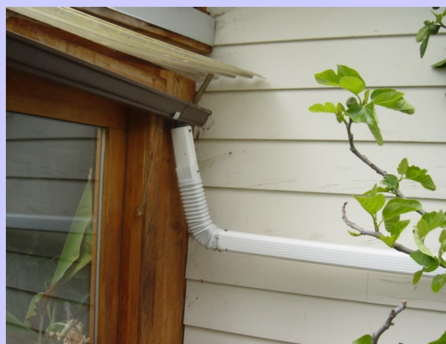
Water flows from roof to tanks
