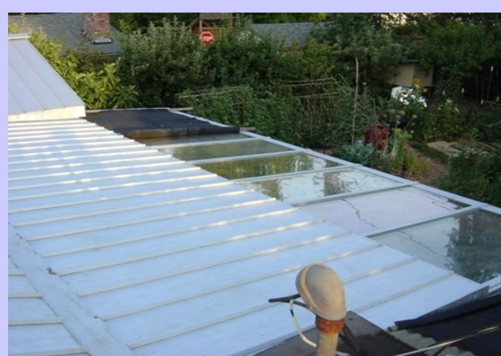
Above the sunroom. Note glass and galvalume roofing.
