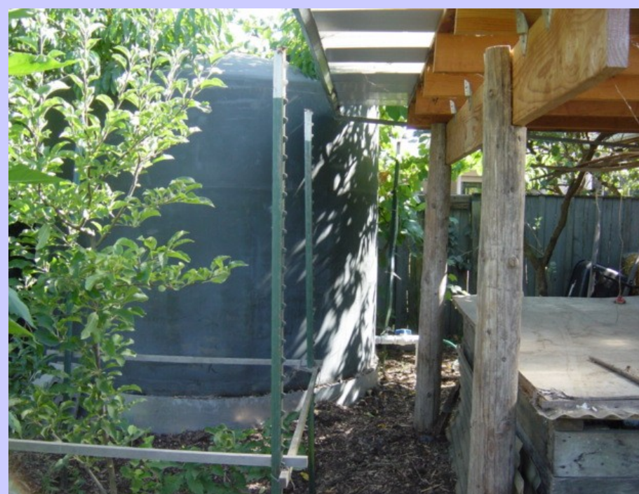
3000 gallon tank in place with the bungalow
